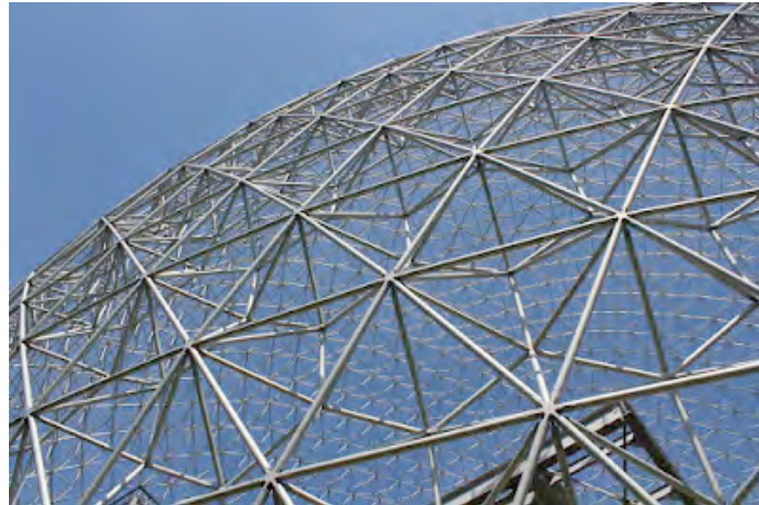
FIGURE 6 Flat triangular segments on the surface of a Buckminster Fuller geodesic dome. A single flat segment is the geometric analog of a locally flat patch in curved spacetime around a black hole; we add local coordinates to this patch to create a local frame. (Figure 3 in Section 3.3 shows a complete geodesic dome with six-sided segments.)
